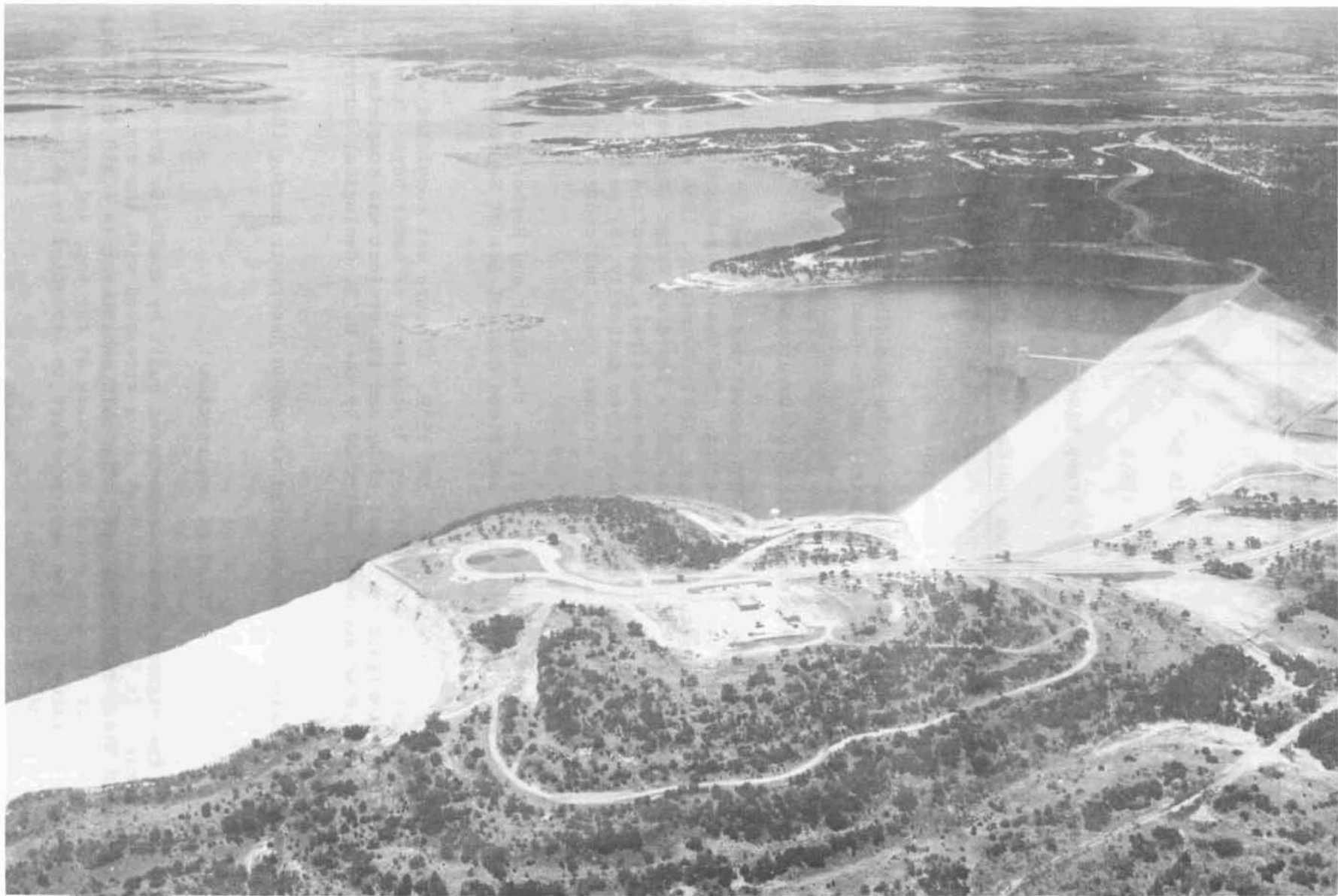
Canyon Dam and Canyon Reservoir. Furnished by U. S. Army Corps of Engineers. Fort Worth District.
