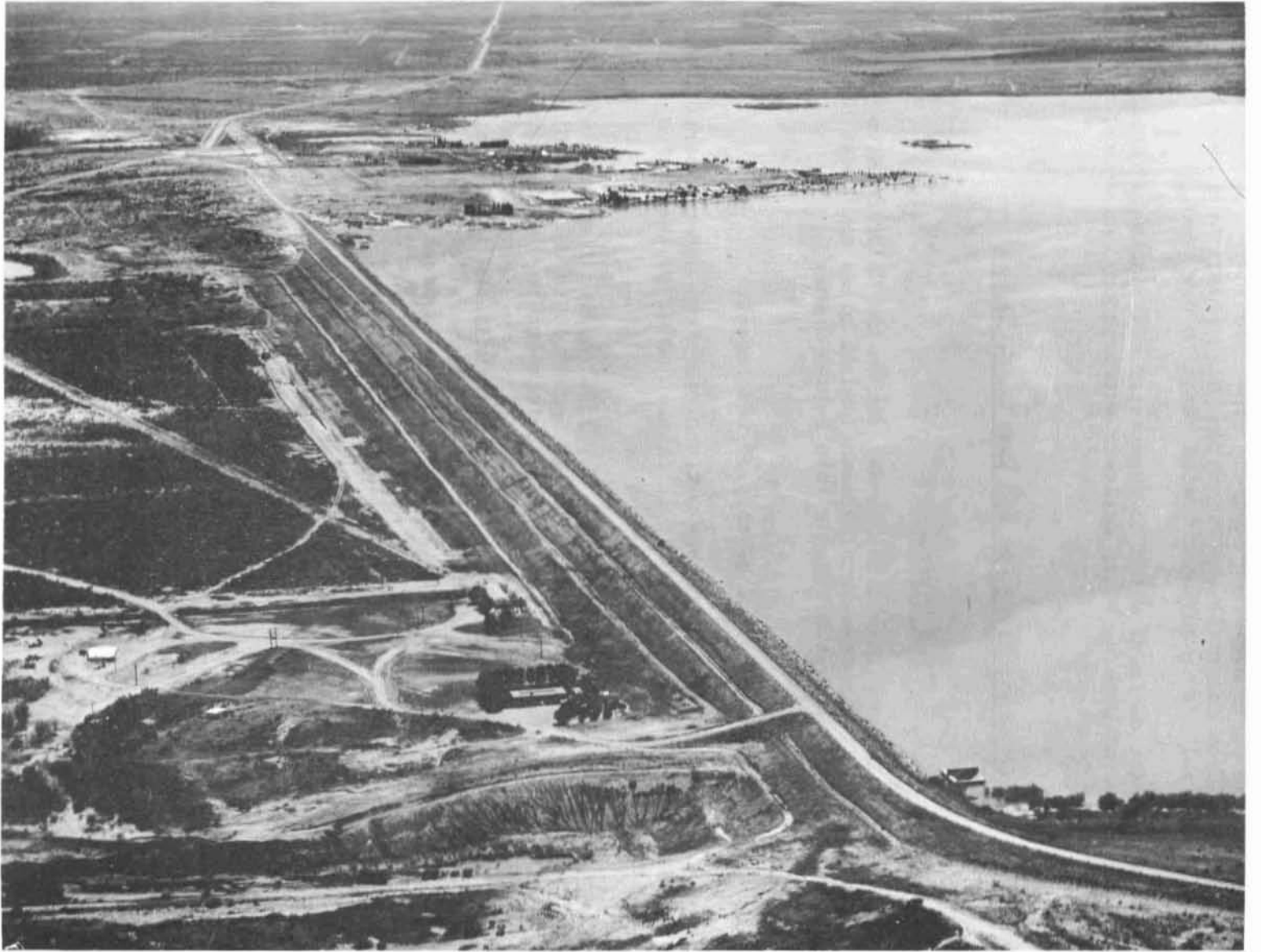
Colorado River Dam and Lake J. B. Thomas. Furnished by Colorado River Municipal Water District.
