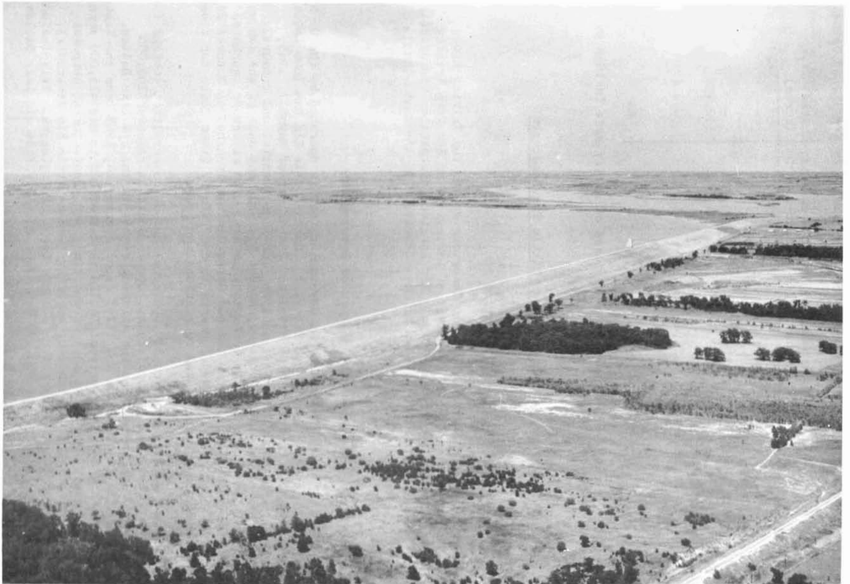
Lewisville Dam and Garza-Little Elm Reservoir. Furnished by U. S. Army Corps of Engineers, Fort Worth District.
