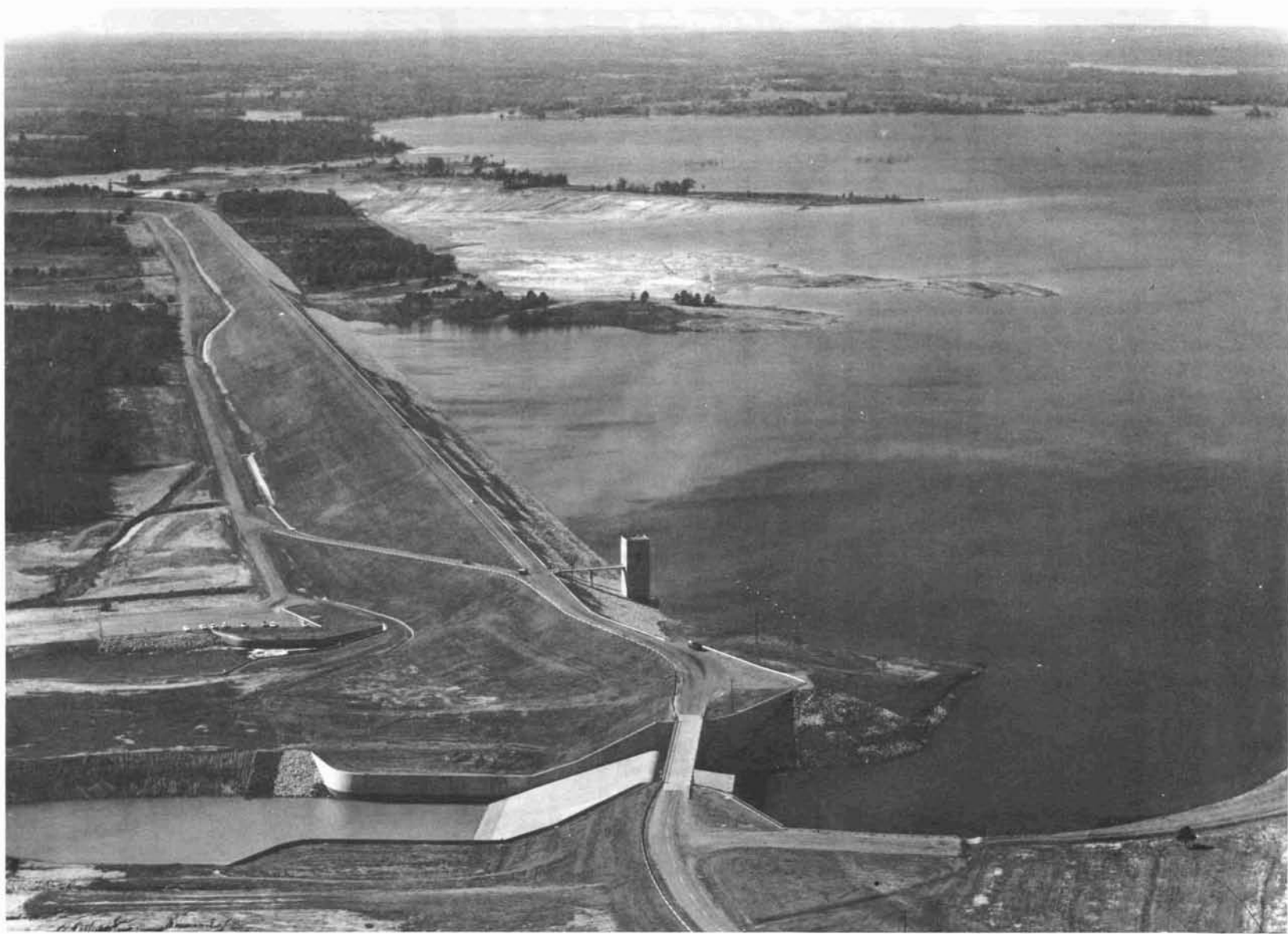
Ferrells Bridge Dam and Lake O' the Pines. Furnished by U. S. Army Corps of Engineers, New Orleans District.
