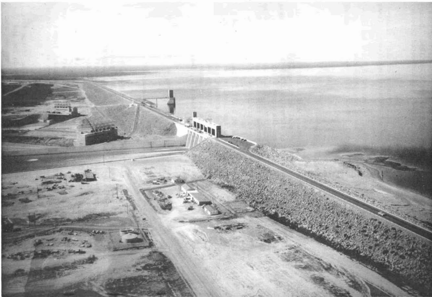
Falcon Dam and International Falcon Reservoir. Furnished by International Boundary and Water Commission, United States and Mexico.
